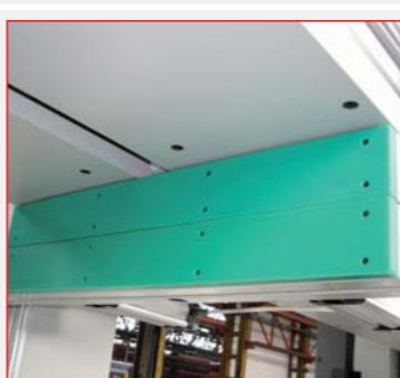
Beams covered with PVC material
